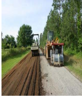
Fig 1: Road reconstruction with FDR
